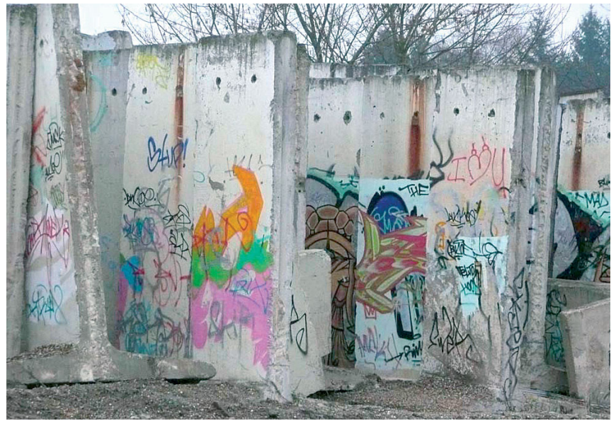
Dismantled wall elements on the Teltow Canal
