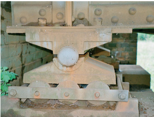
Typical historical bridge bearing
