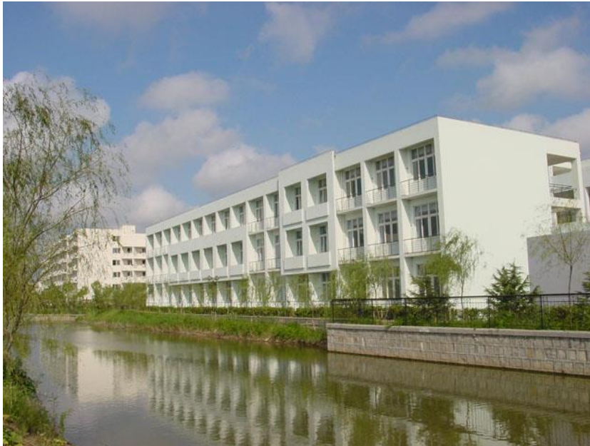
Building of a Lab
