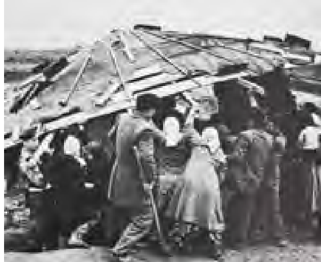
Rebuilding of gecekondus [unknown photographer]
