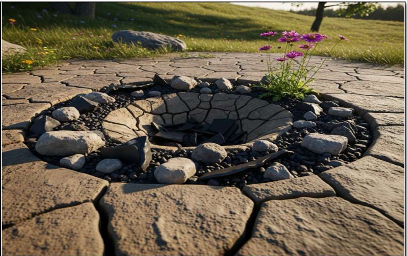
Figure 3 Displacement: Fractured Ground
