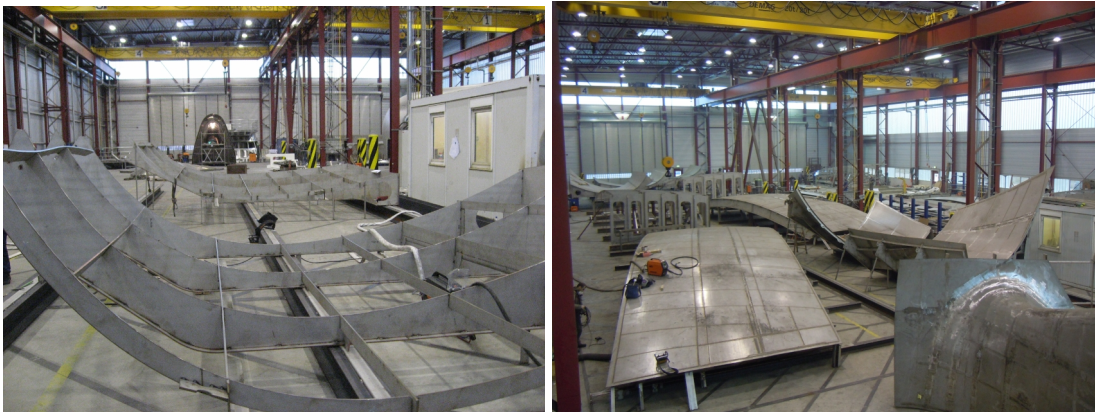
Fig. 8 Assembly of stainless steel sheets in the factory
