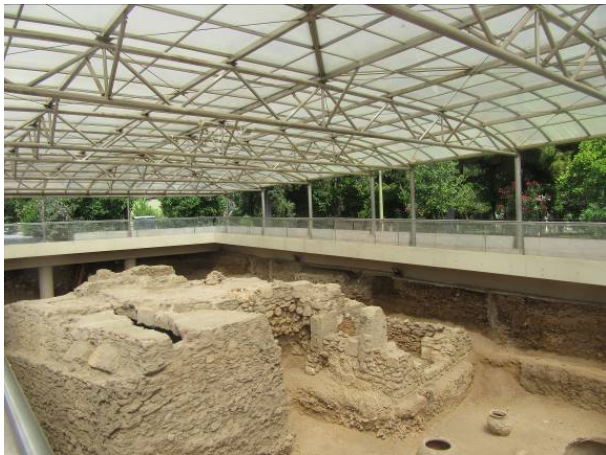
Fig. 8 Truss roof, near the Syntagma square in Athens, Greece [8]
