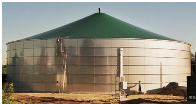
Figure 1: Closely ring-stiffened cylinder (l., [1]) and widely ring-stiffened tank (r., [2])
