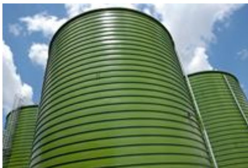
Figure 1: Closely ring-stiffened cylinder (l., [1]) and widely ring-stiffened tank (r., [2])
