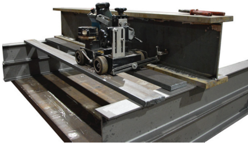
Figure 4. Test setup for the manufacture of welded I-girders, MAG welding tractor.
