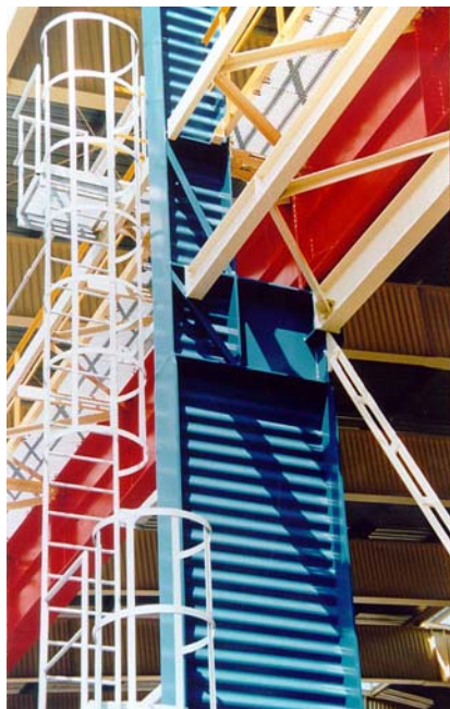
Fig. 3. Crane way column
