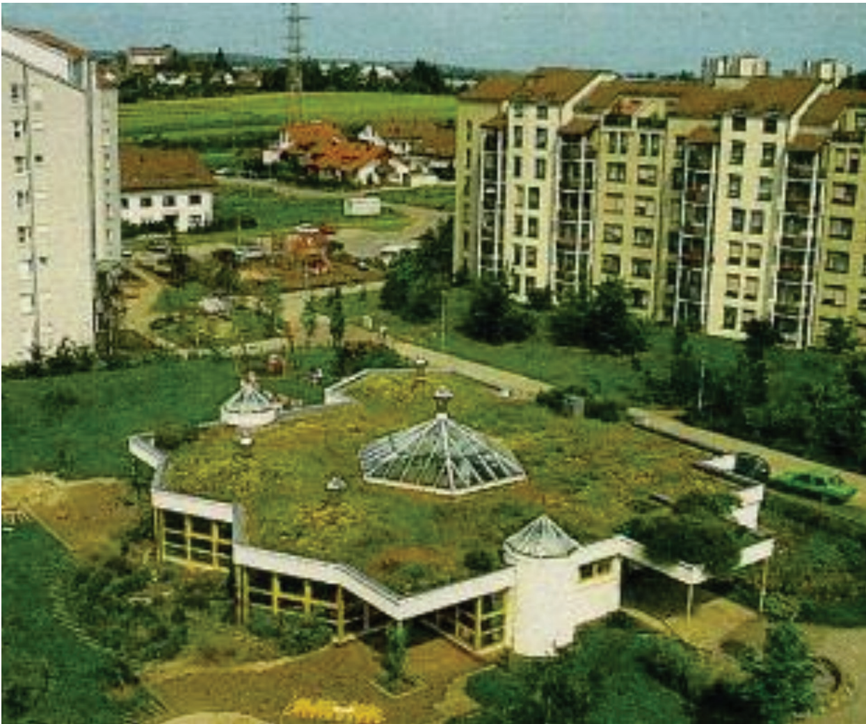
Fig. 2.16. Example of green roofs as a measure for delayed rainwater runoff and improvement of the microclimate (evaporative cooling) [Source: Department of Urban Technical Infrastructure, BTU Cottbus Senftenberg]
