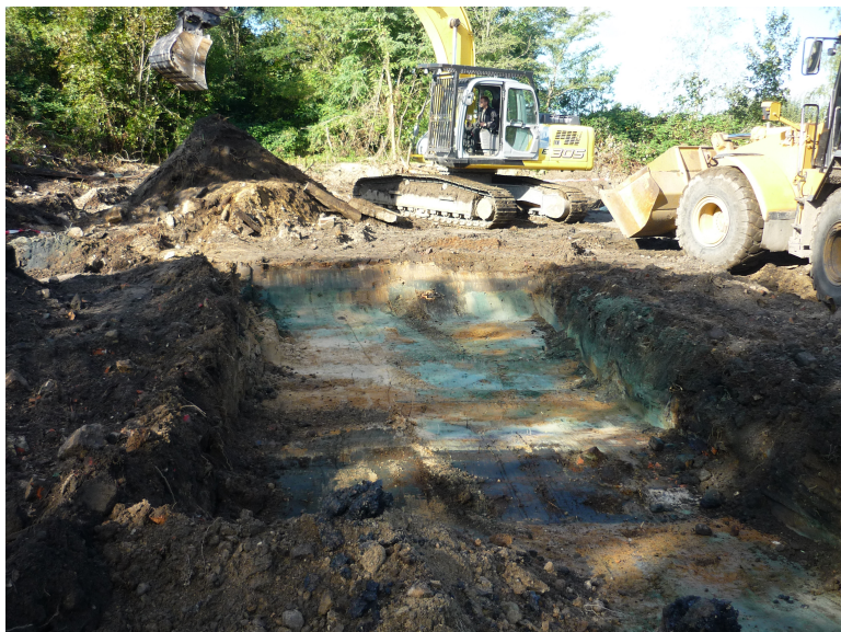
Picture 3: Remediation operations: removal of the contaminated top soil (photo made by Dr. Repmann).
