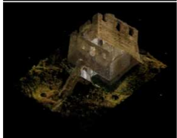
Figure 6: Point cloud of the Torre Cavallara survey, near Catanzaro
