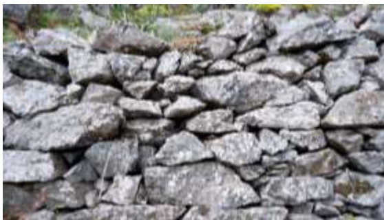
Figure 1: Detail of the connection system of a dry stone structure. Photo by the author.
