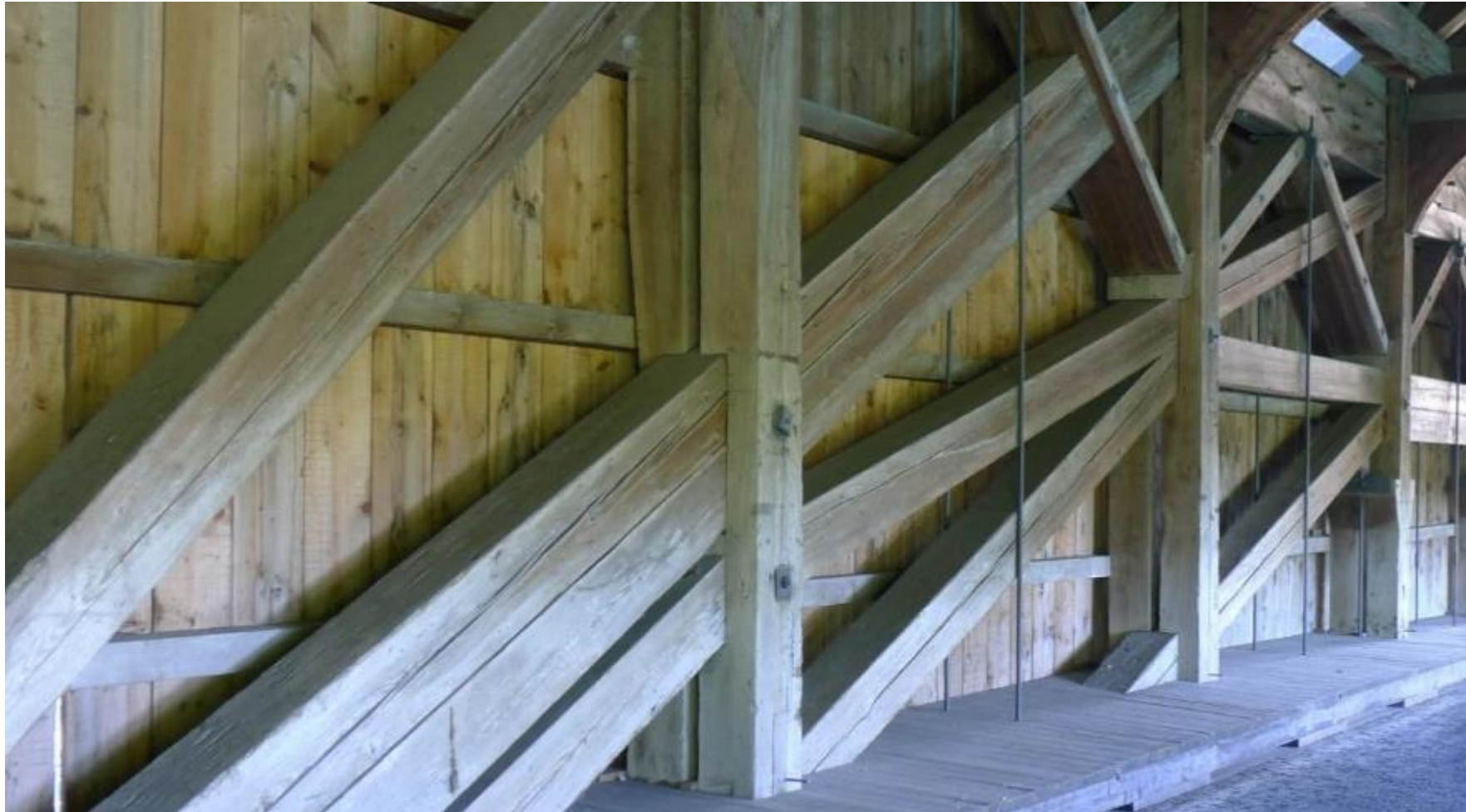
Historische Holzbrücke (D. Wendland)
