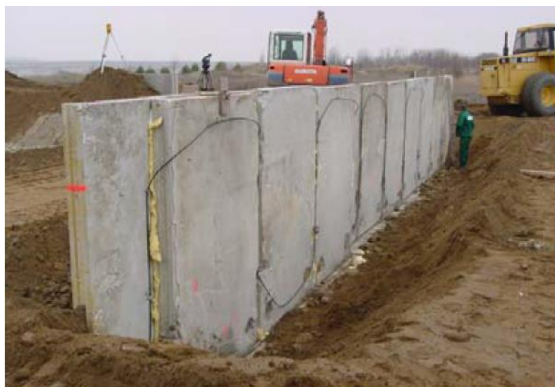
Fig. 7.11: Installation of the temperature cable
