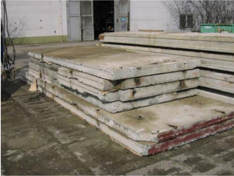
Fig. 6.4: Interim stored ceiling panels in the outdoor area
