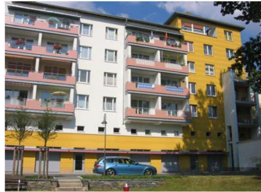
Fig. 3.14: Residential building with an underground car park in Plauen (Planning: Prof. W. R. Eisentraut)
