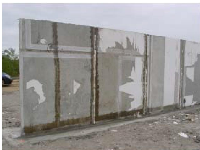
Fig. 7.9: Inner sealing; top view and in the construction phase
